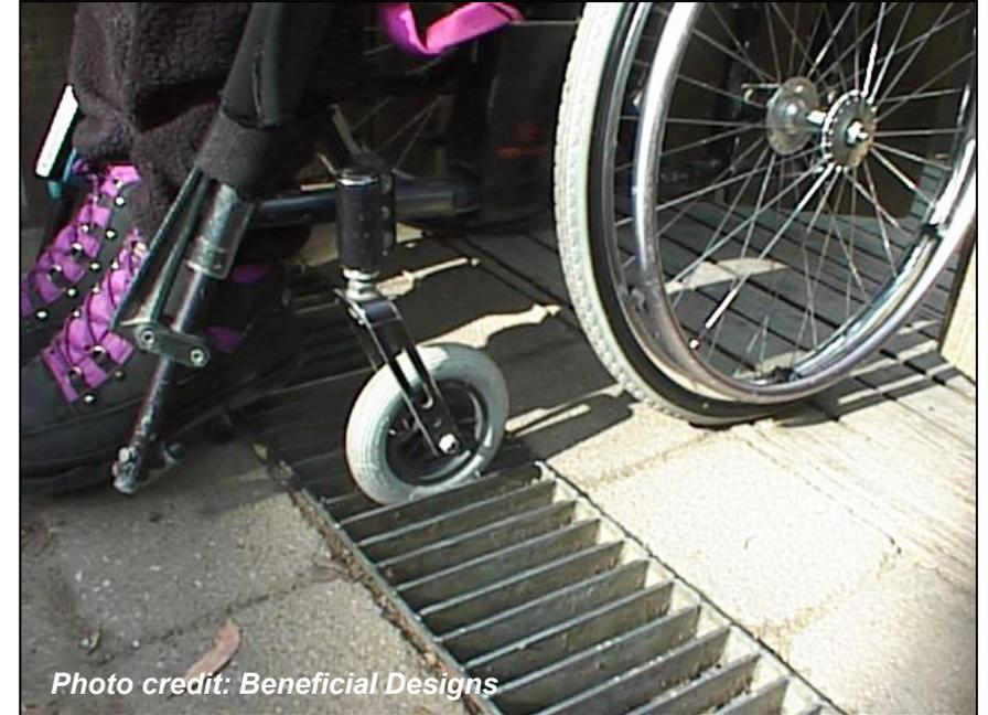
**R302.7.3 Horizontal Openings** - . . . Shall not permit passage of a sphere no more than 0.5 in. Elongated openings shall be placed so the long dimension is perpendicular to the dominate direction of travel.
