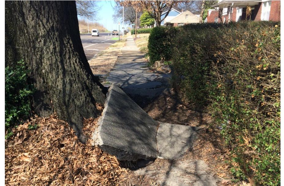
**R302.7.2 Vertical Surface Discontinuities** – Vertical surface discontinuities shall be 0.5 in. maximum. Vertical surface discontinuities between 0.25 in. and 0.5 in shall be beveled . . .
