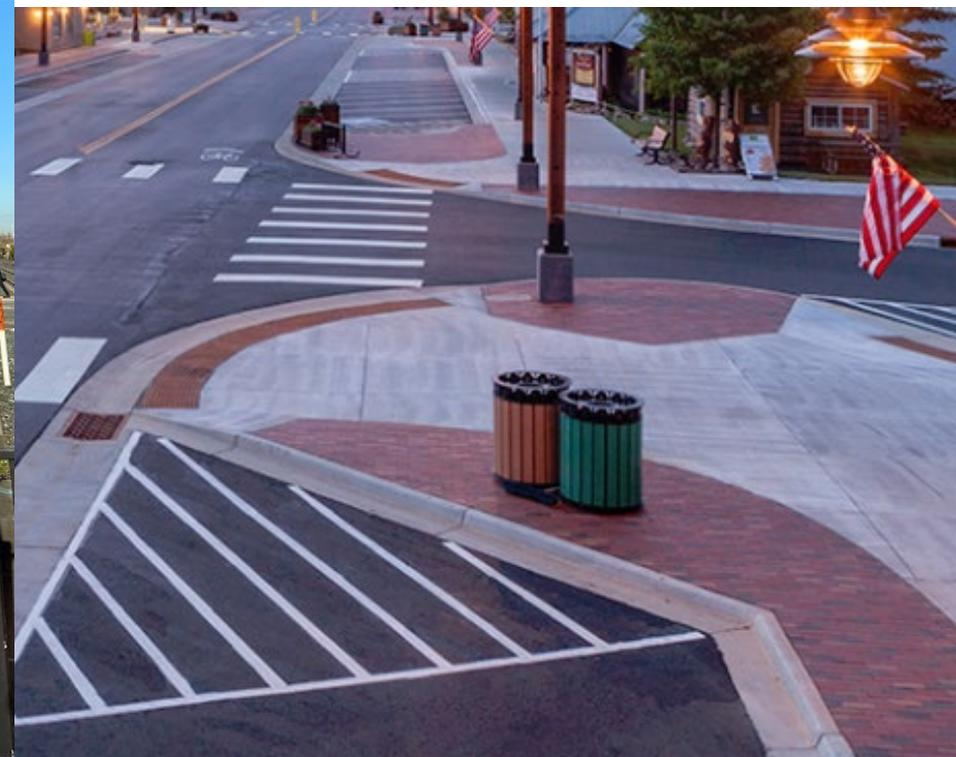
Sidewalk surfaces shall be firm, stable, and slip resistant.
