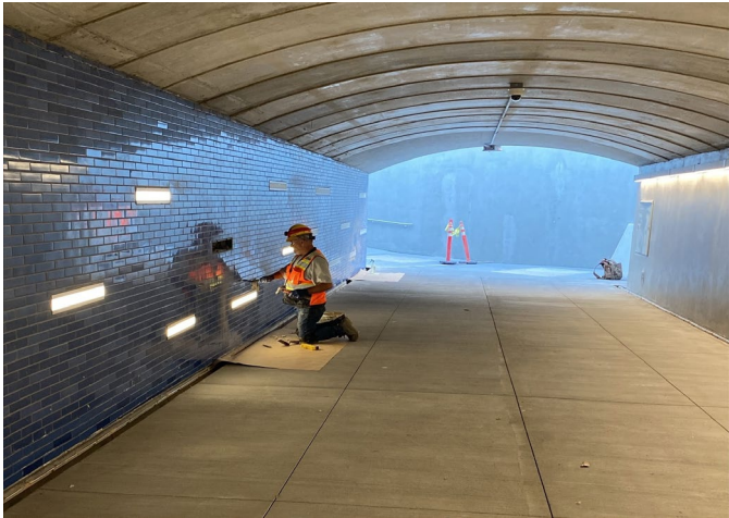
Photo 3 - Ped Underpass looking east
