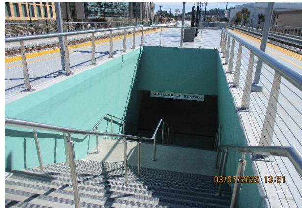
Photo 4 - Stairs Paint Touchup at Hillsdale Station
