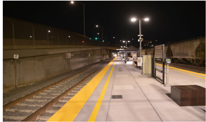
Photo 2 -New platform looking north MT-2
