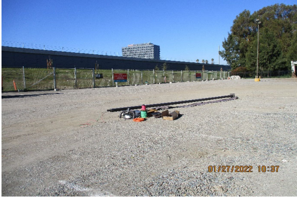
Photo 1 - 25th N Yard Lighting Pole
