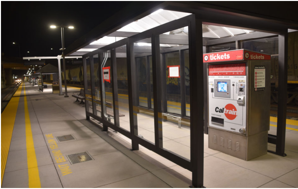
Photo 1 - Shelter with ticket machine
