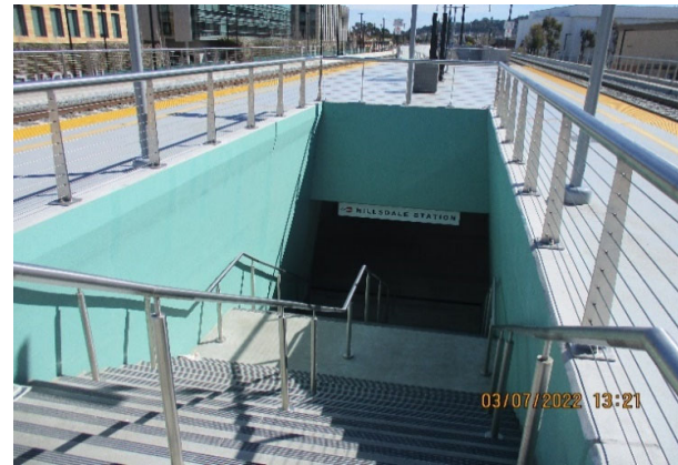
Photo 4 - Stairs Paint Touchup at Hillsdale Station
