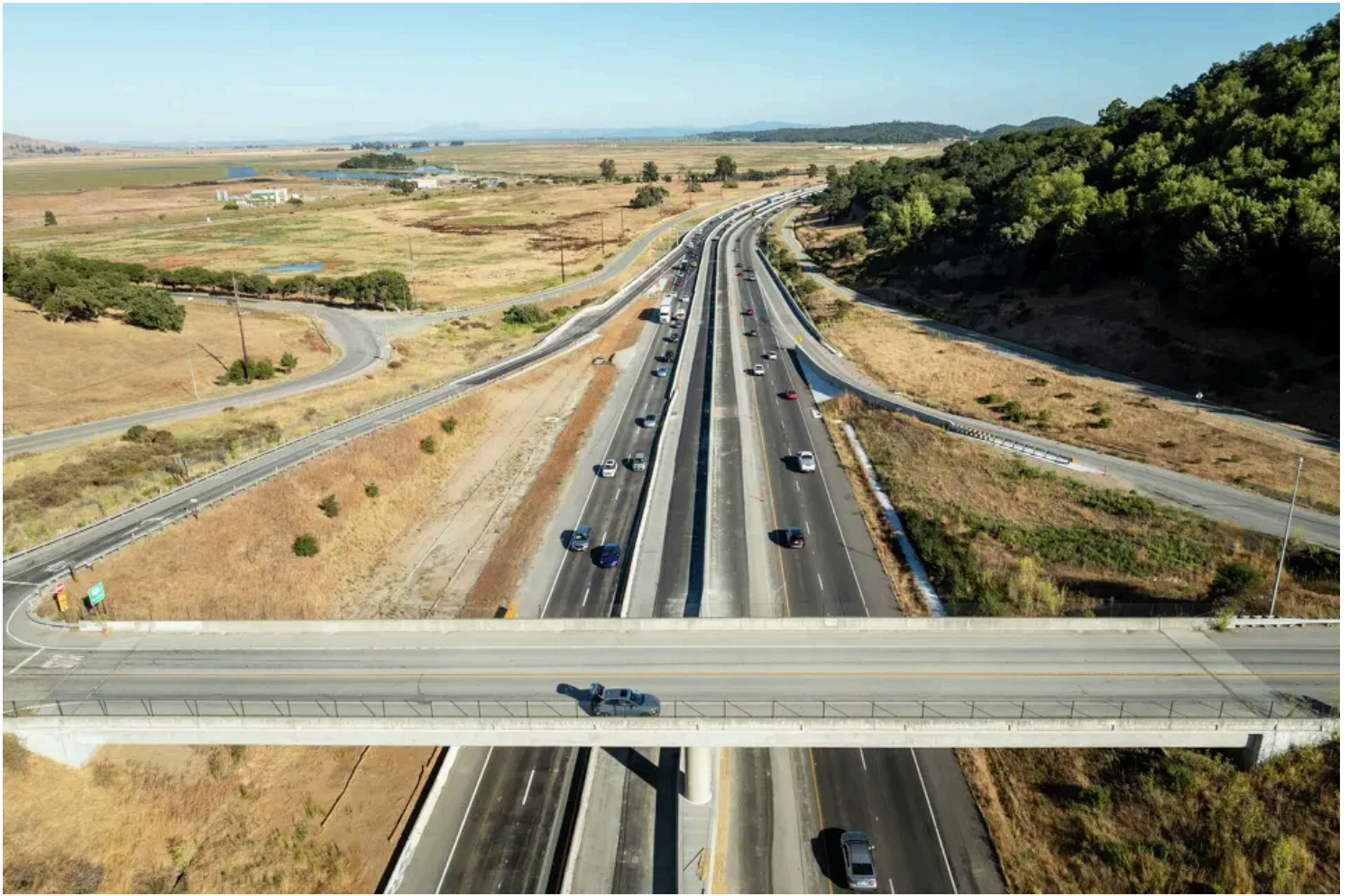
Aerial views of the new lane construction along Highway 101 near Petaluma, in August. The widening of the road took decades to finish, but now some commuters say it has made traffic worse during rush hour periods.
