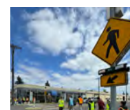
Rectangular Rapid Flashing Beacons (RRFBs)
