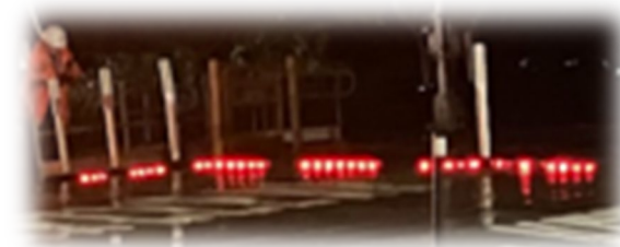
Delineators & Solar Markers @ night.
