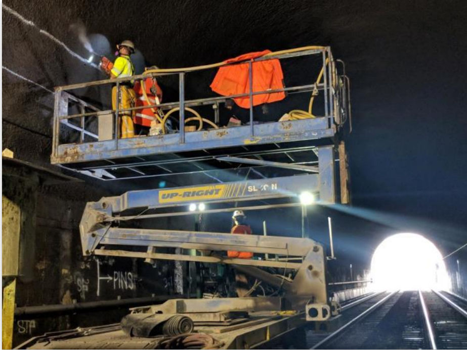
Dry Fix Pin Installation
