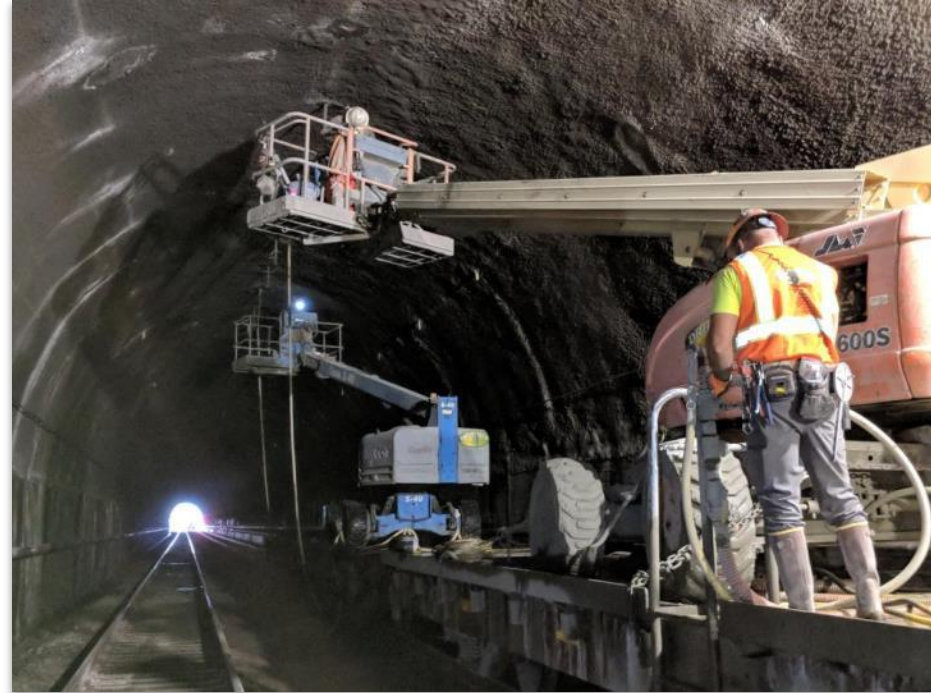
Grouting Operation
