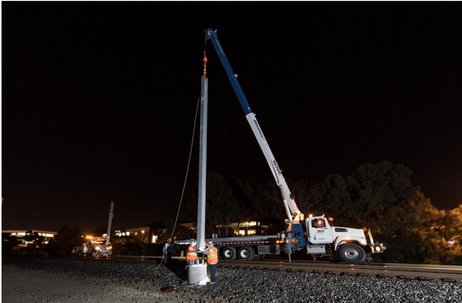
OCS pole lifted off flatbed truck
