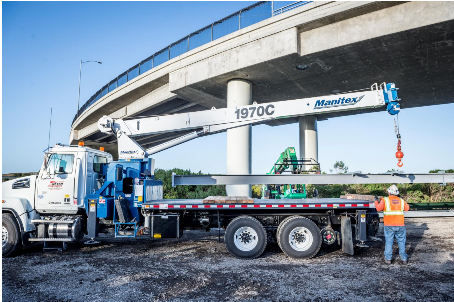
OCS pole on flatbed truck
