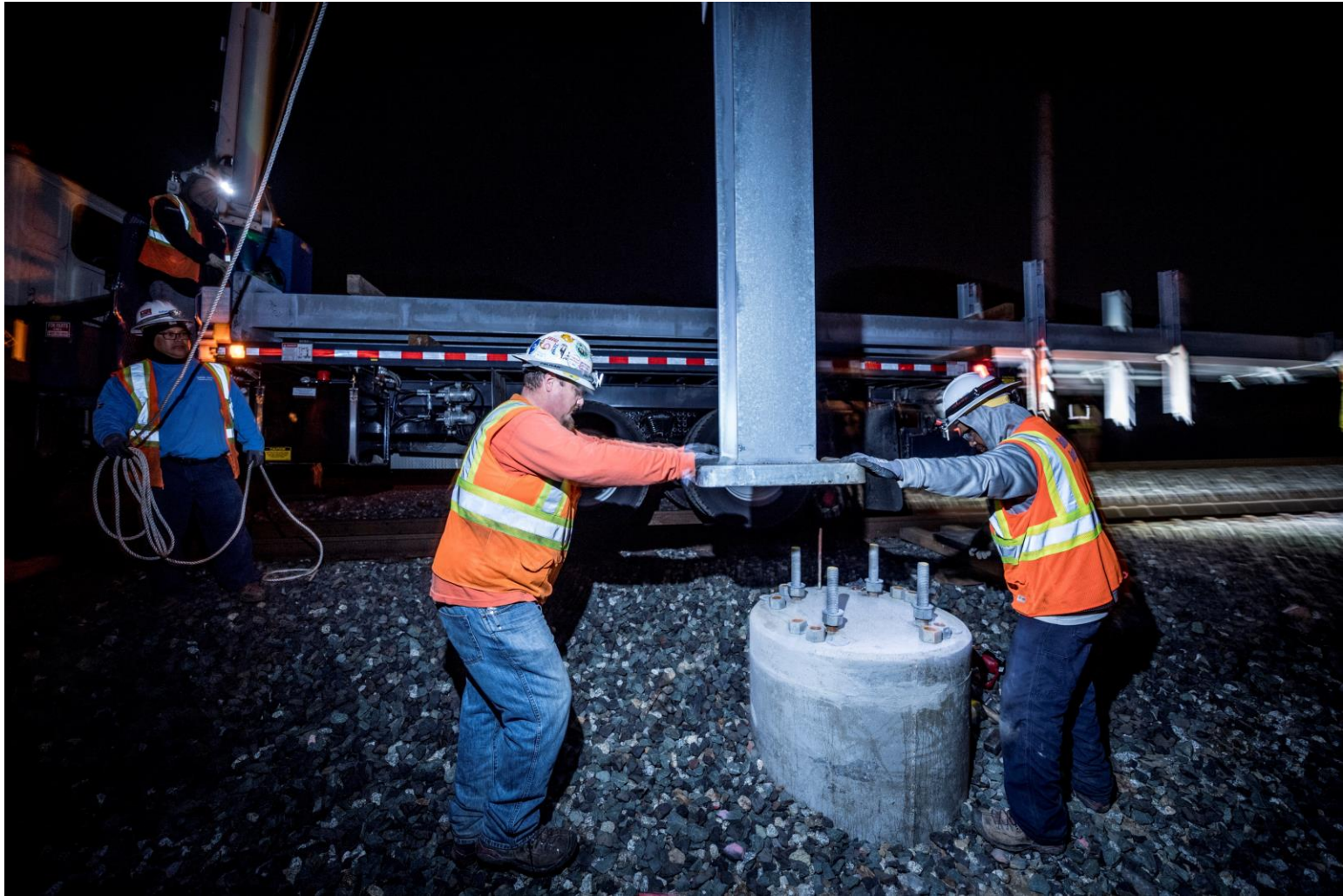
Crew placing OCS pole on foundation
