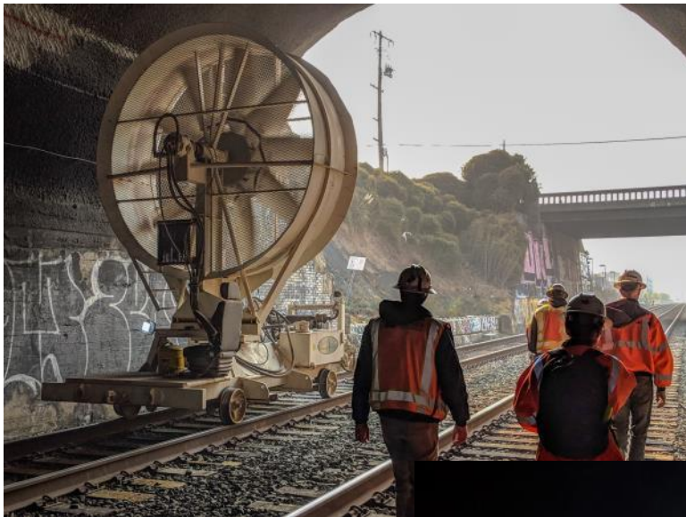
Fan used to maintain airflow during notching
