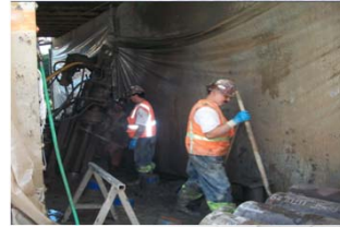
Foundation Improvements completed in 2011
